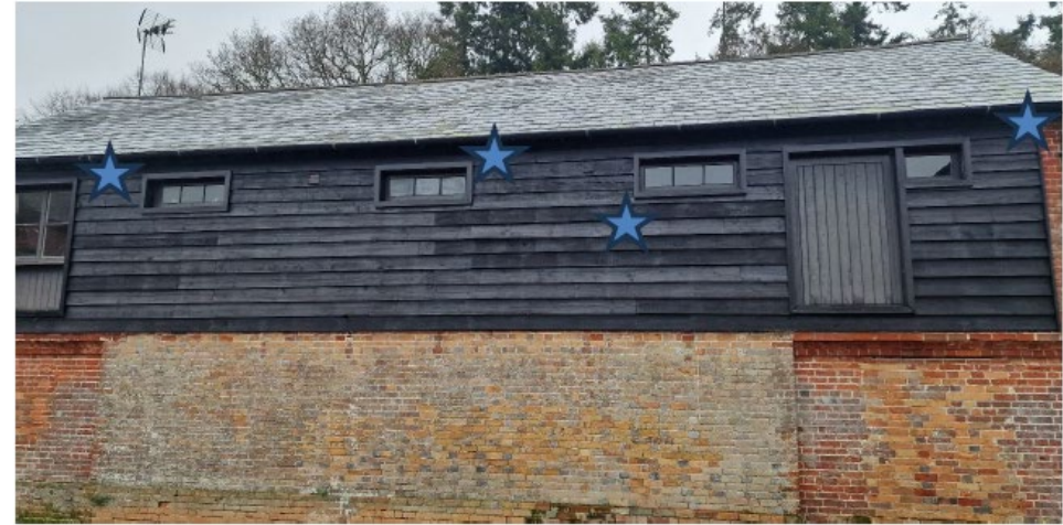
Figure 5: Showing areas where bats emerged southern elevation
