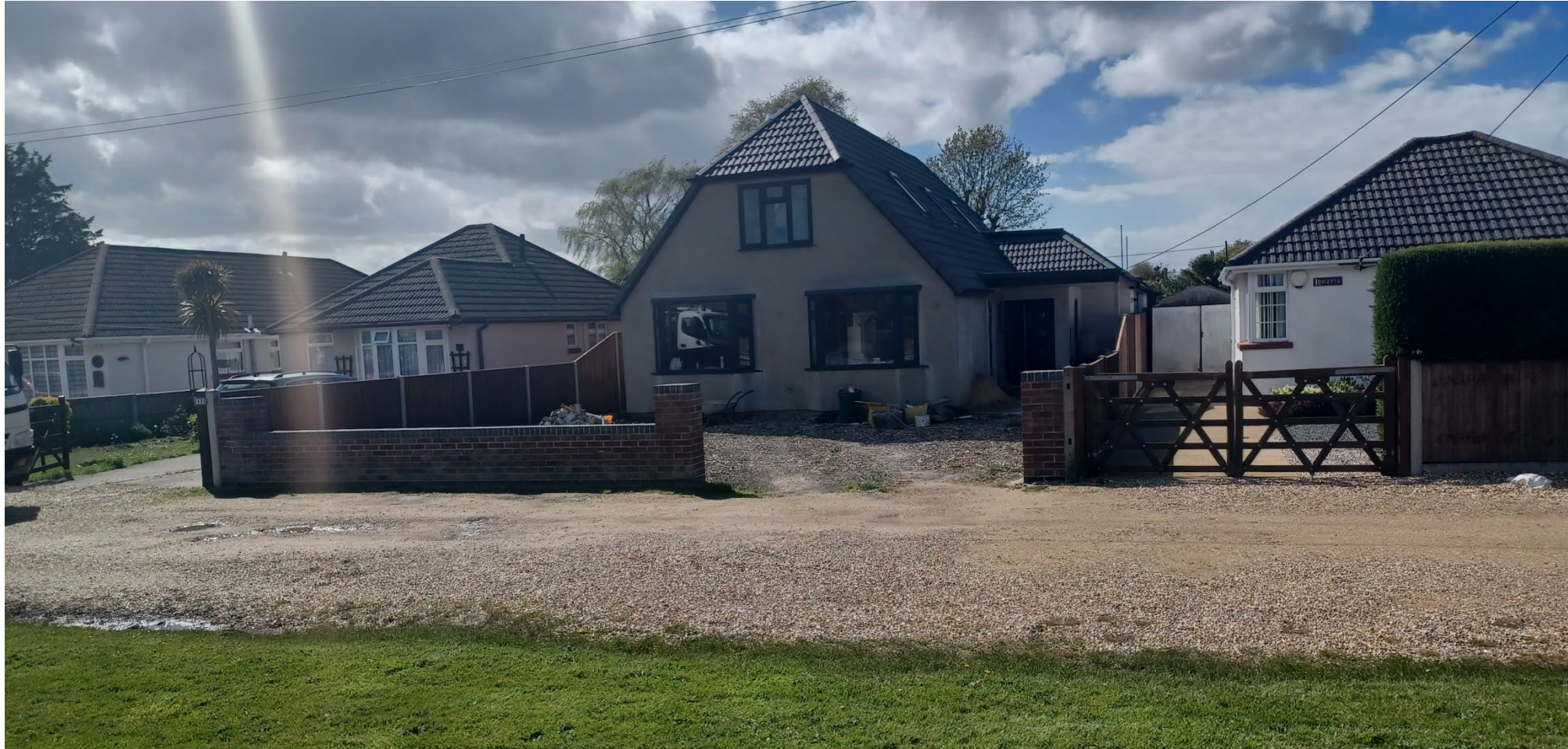
Wider shot of frontage, including accessway
