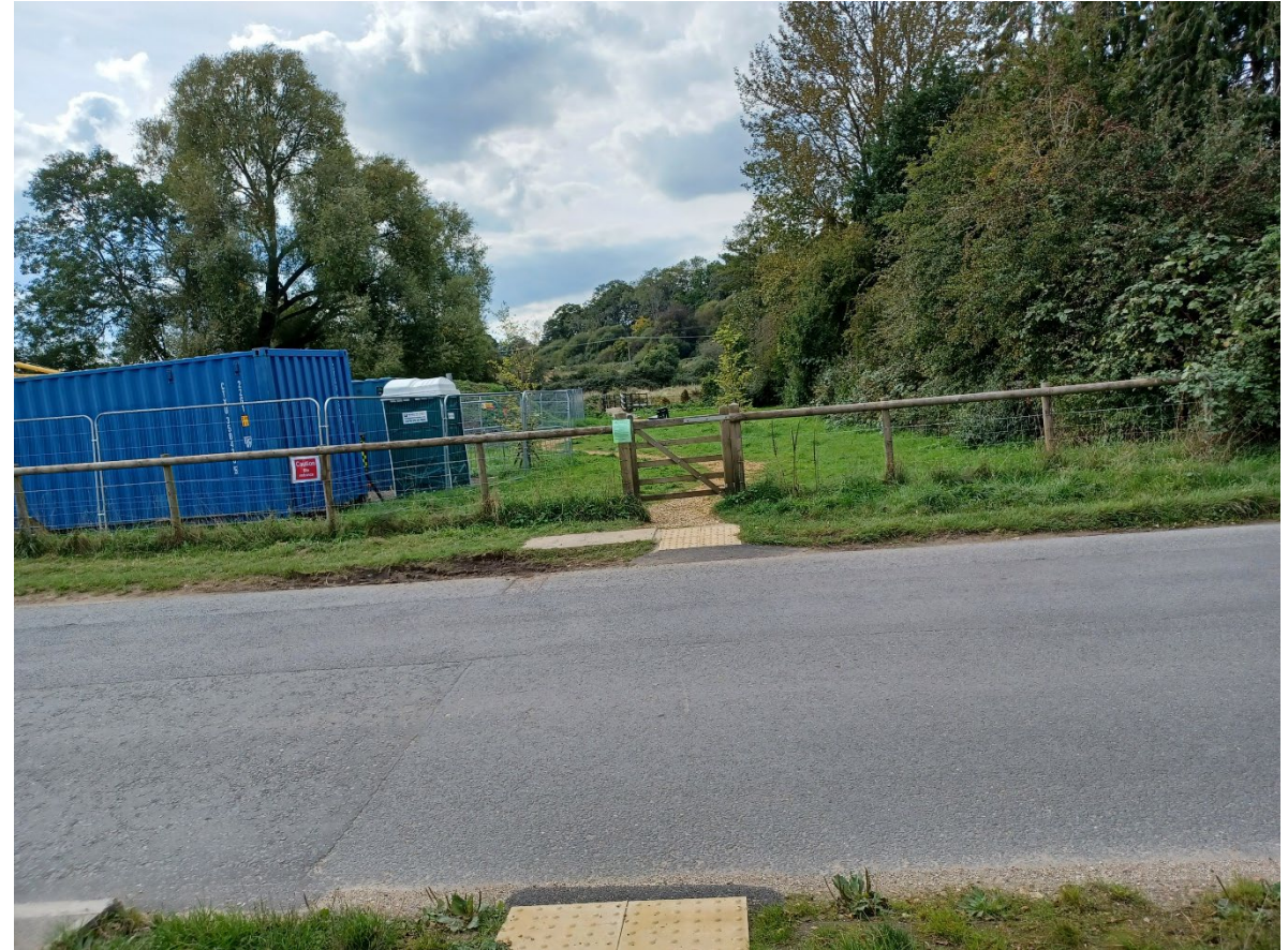
Site of proposed temporary access
