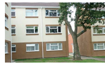
Flats on the North Milton Estate after refurbishment
