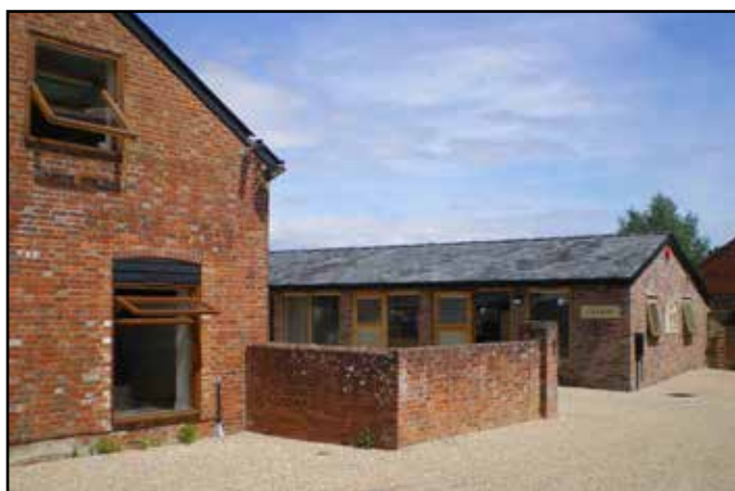
Office development at Efford Farm
