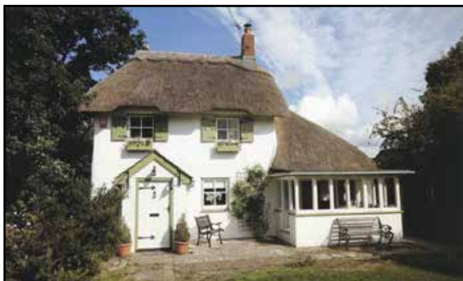
Swan Cottage-(formerly Yeovilton Lodge and Everton Post Office) a traditional cob cottage (Listed grade II) *5
