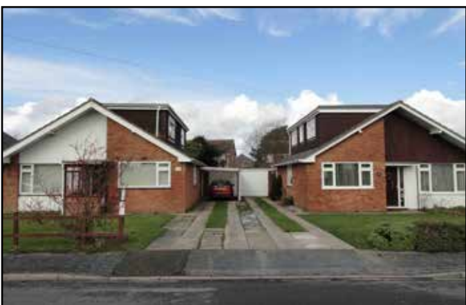
Impact of roof conversion at Pinewood Estate
