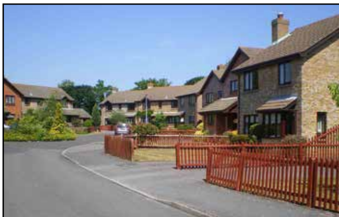
Brickwork and limited landscape at Laburnham Drive
