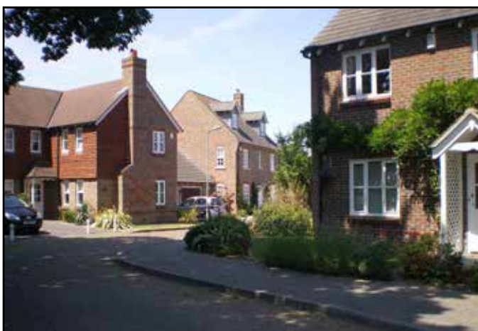
Finishes & landscape can soften the impact of development
