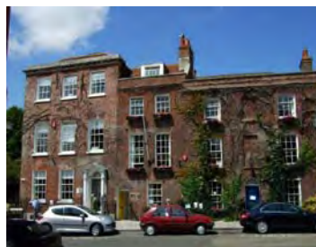
Fig 1.9 Classical rules of proportion allow a very tall three storey building to sit quite comfortably within scale of the street. The hierarchy of window proportions, with smaller windows on top floor and the parapet wall holds the facade allowing the purely functional part of the roof to recede behind. The building width and pattern of windows and doors reflects the rhythms of the street set up long years before, as burgage plot frontages.
