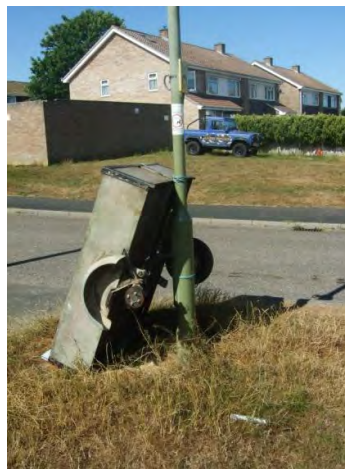
Fig 9.14 Open space is plentiful but underutilised or occasionally misused – it makes rather monotonous play space, and although most spaces are at least green all year round, they often provide scant visual amenity.
