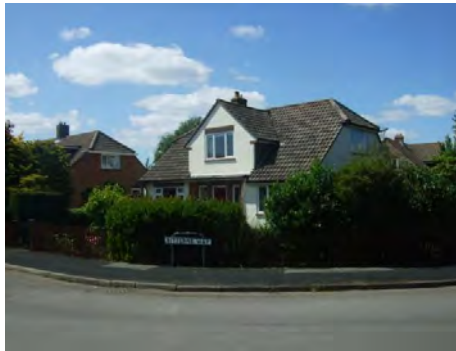
Fig 6.4 Most of the dwellings in the western half of the area were built as 1½ storey chalet bungalows exhibiting a similar form with half hipped roofs and central gable.
