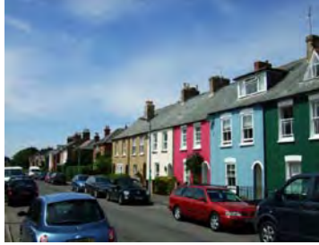
Fig 1.18 Varied terraces, detached and paired dwellings in the Western Road part of Six Acres. Articulated skyline in rhythm with the plot divisions, eaves lines are fairly consistent, and various small set-backs together with a fashion for painted facades allow personalisation.
