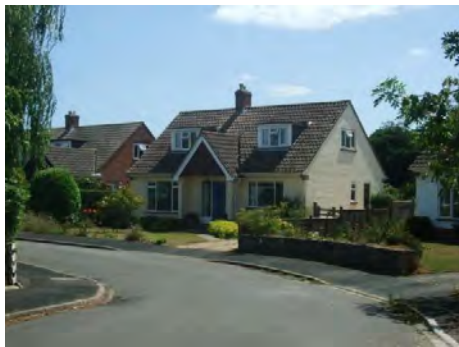
Fig 6.5 Variations on the chalet bungalow form with a prominent gable over the front door and proportionate dormer windows set back into the roof plane.
