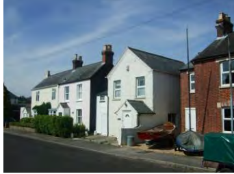
Fig 5.13 Spring Road - part of the phase 2 'grid' - A cluster of traditional rural dwelling types suggestive of a village centre, two recent buildings have underpinned this effect using traditional materials and details within similarly proportioned cottages.
