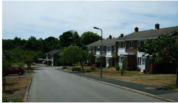
Fig 7.17 Rowans Park: Open plan layout of smart terraced dwellings in a communal garden and parking court setting. The group is introverted behind tall fences and hedge, and enjoys considerable communal open green space which forms the all-important backdrop.
