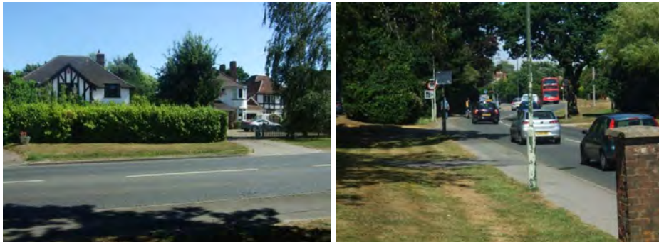
Fig 9.4 Varied suburban houses in large garden settings and the green verges that make up the 'green corridor' character of Milford Road.
