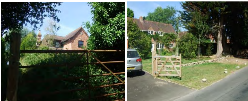
Fig 10.9 Scale, set-back and setting is important to allow each of the buildings to nestle comfortably amongst the taller trees or behind the hedgerows seen from the lane.
