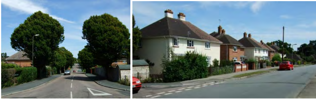
Fig 7.11 Highfield Avenue is framed, to either side, by the neat forms of two typically English groups of unspoilt semi detached houses.
