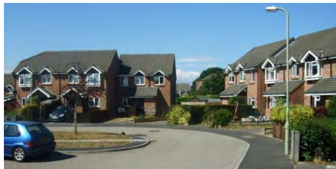
Fig 9.9 Deneside Copse consists of a striking group of consistent houses with decorative 'mini' gables over upstairs windows. On the western edge they surround a play area and greenspace. Front gardens are often in full use for garden activity from vegetable plots to paddling pools as well as the inevitable car spaces.
