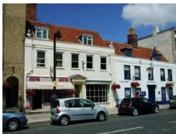
Fig 1.8 Combination of traditional roofscape with more classical Georgian rules of proportion applied
