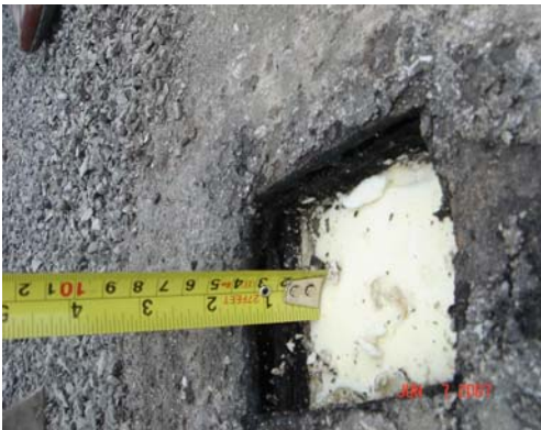
Confirming Depth of Membrane Build Up
