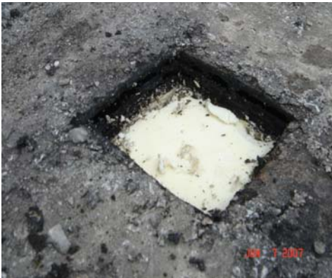
Confirming Roof Build Up
