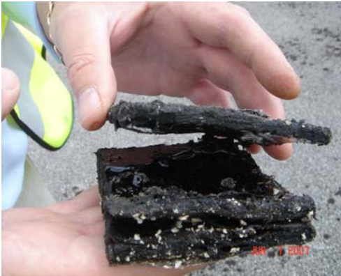
Further Confirmation of Existing Roof Build Up
