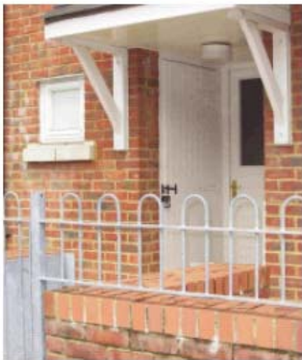
On the same development whilst the design intention is good the execution doesn't meet expectation. Doors on the front of the enclosures might have produced a better end result.
