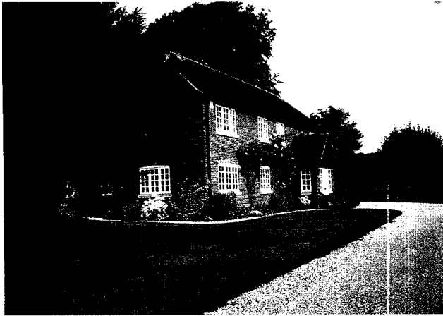
'Cross Trees' a recent rebuild to replace a listed building burnt down
