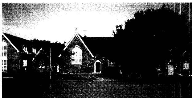
Village School with New Extension
