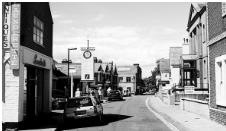
New Street - a more fragmented piece of townscape, with opportunity for redevelopment and improvement
