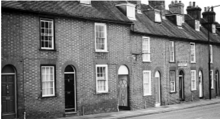
Stanford Road - brick listed buildings with grey-blue headers used throughout
