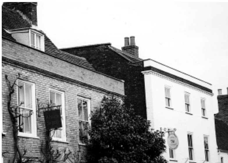
Parapets in brick and render topping the front elevations on St Thomas's Street
