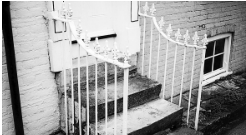
Stone steps and original railings on Nelson Place. Original railings are now rare
